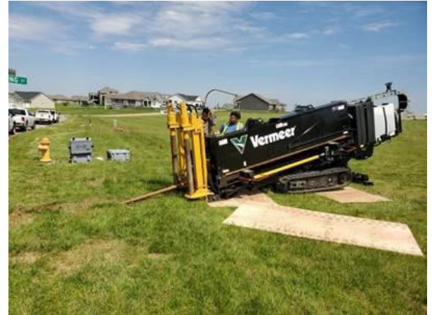
Construction crew laying fiber in the City of Pella
